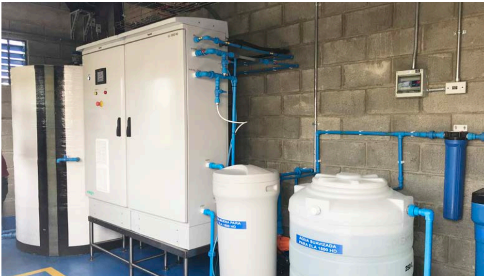
Envirolyte ela1800HD set for 5000ppm for public water treatment
